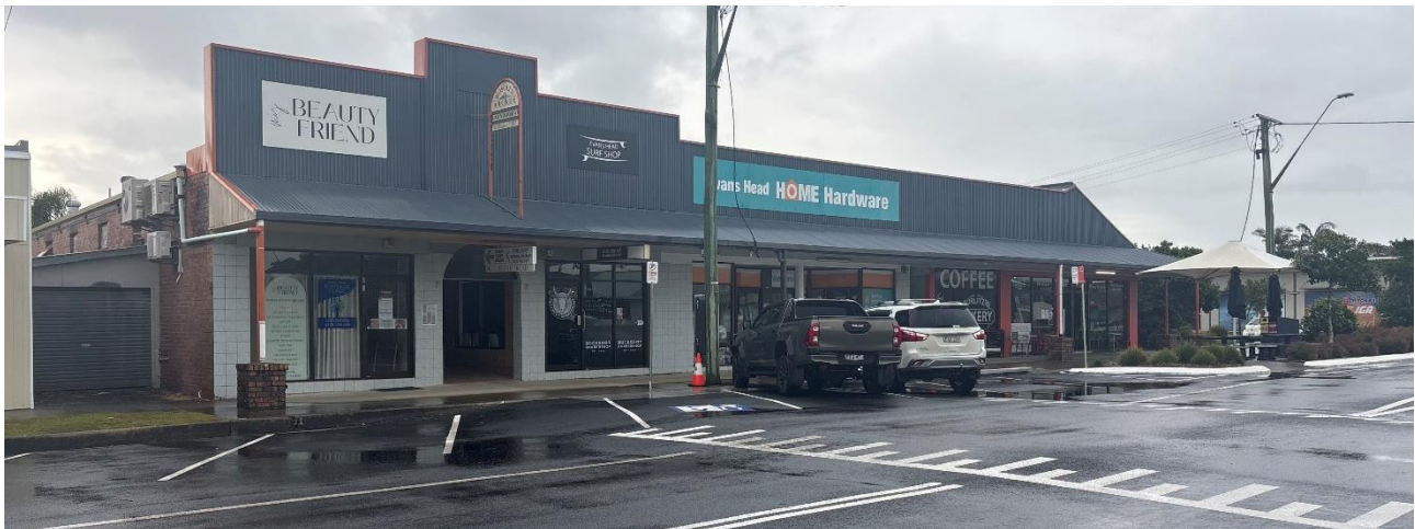
Image 1 – EV Charging Station installed
