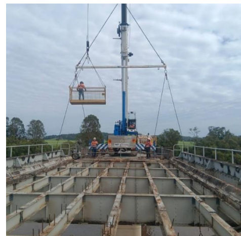
Removing the old deck on Broadwater Bridge
