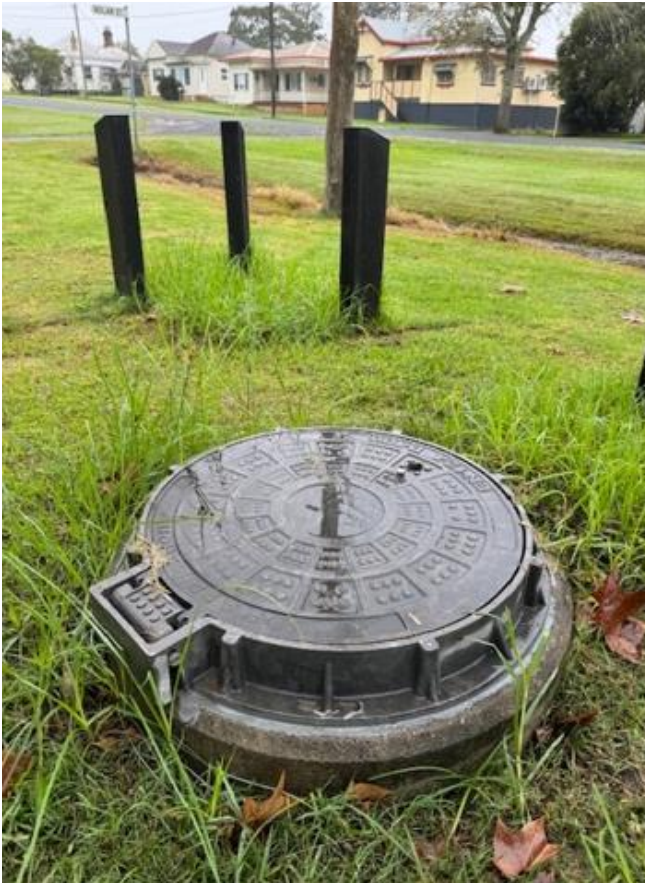
Image 6 – New sewer manhole lid Windsor Park
