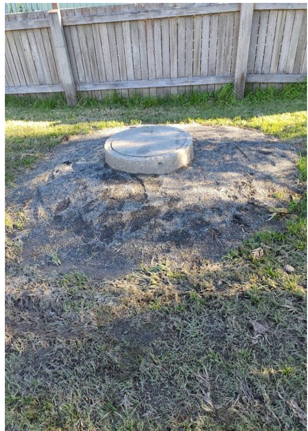
Image 7 – Raised sewer manhole in Church Lane
