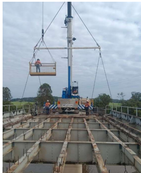
Broadwater Bridge deck being removed for replacement
