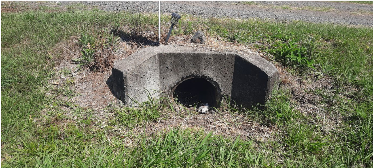
Plate 5.3 View west of concrete pipe culvert within the site
