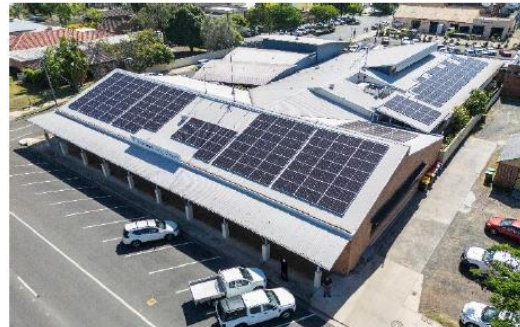
Solar panels on Casino Administration Building
