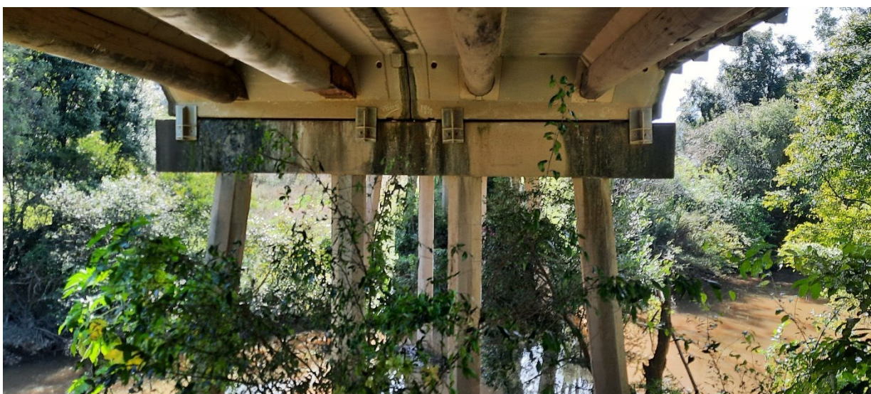
Plate 2.4 View to the north-west, underneath Deep Creek Bridge
