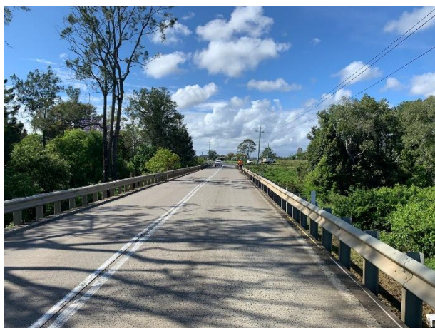
Looking south along the existing bridge deck
