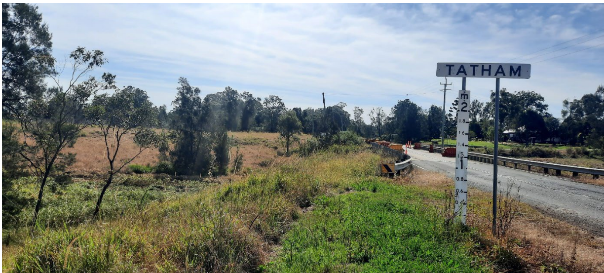
Plate 2.1 View to the north-west of Spring Gully Bridge
