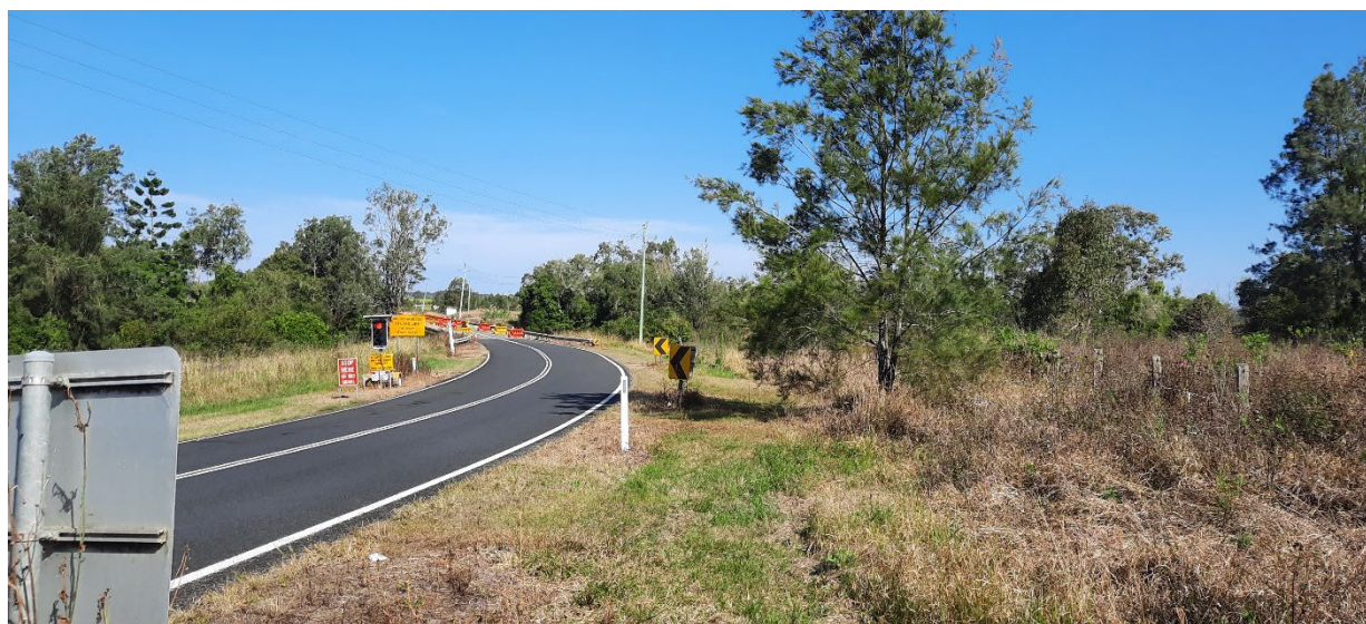
Plate 6.8 Casino Coraki Road - North of Deep Creek Bridge
