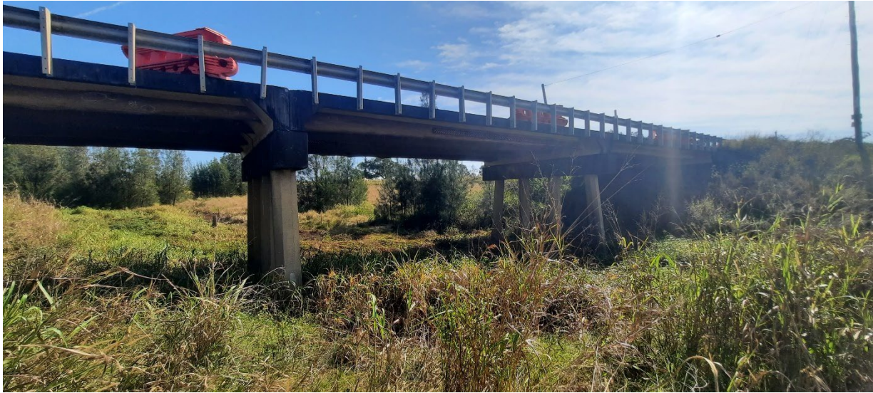
Plate 2.2 View to the east, underneath Spring Gully Bridge
