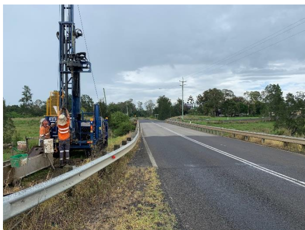
Looking north along the existing bridge deck. Rig setup at BH5.
