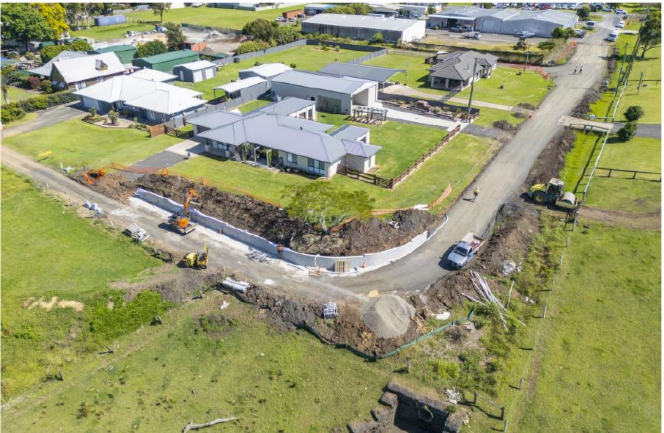
Image: Construction works underway for Country Lane Road reconstruction
