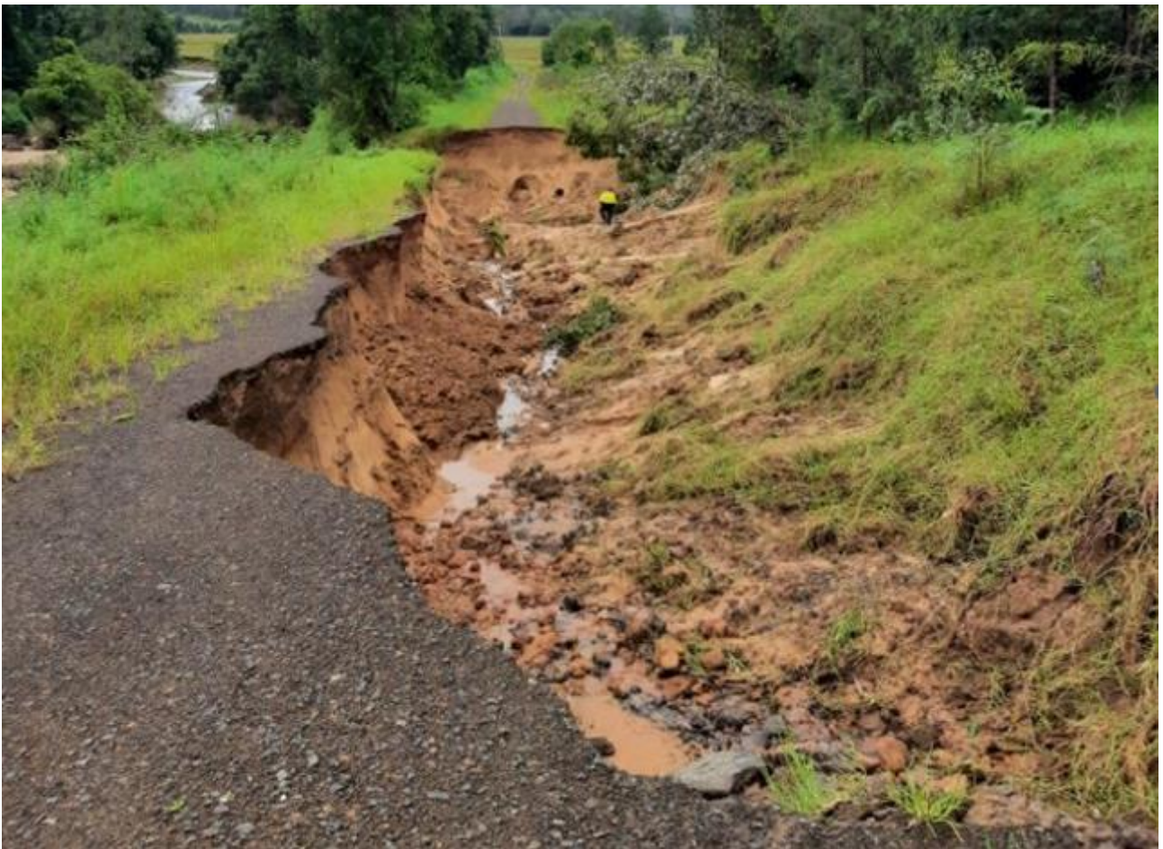
Image 2: Upper Cherry Tree Road landslide.
