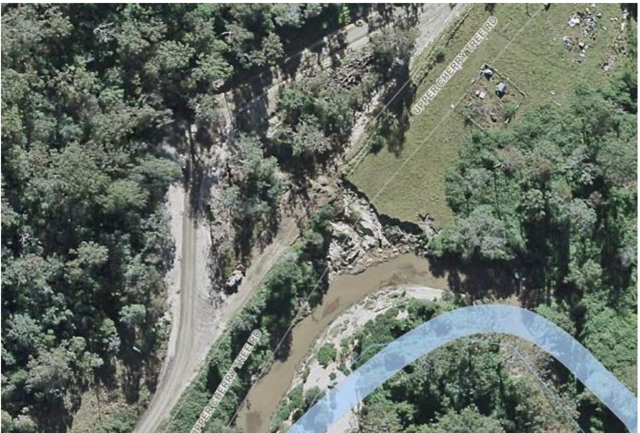
Image 3: Upper Cherry Tree Road post flood aerial imagery of the slip.
