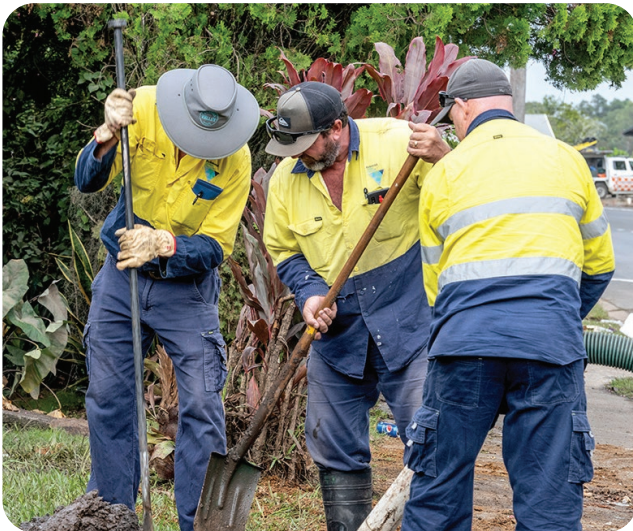
Council's water team carrying out urgent repairs after the 2022 floods.
