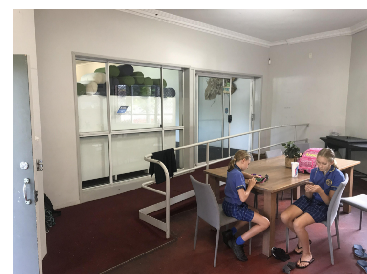
03 EXISTING RAMP UP TO EXISTING MULTI PURPOSE ROOM
