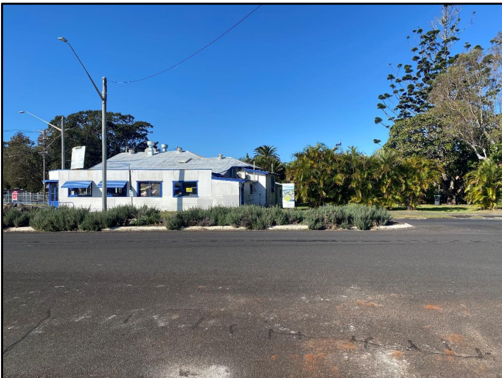
Plate 4: View of subject site from Elm Street frontage
