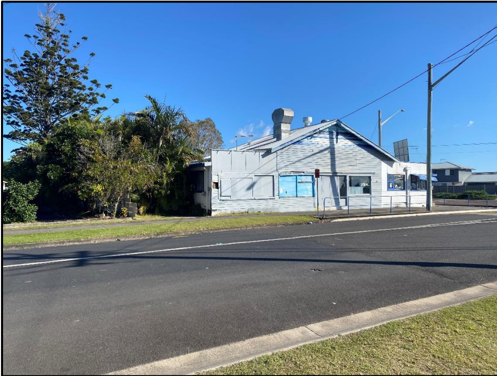
Plate 3: View of subject site from McDonald Place frontage
