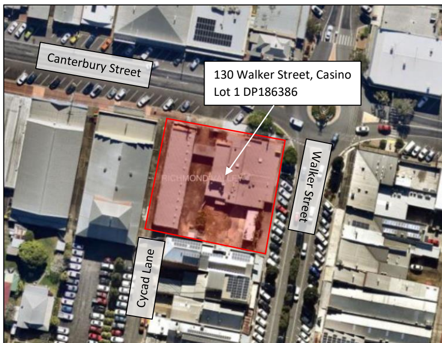
Plate 1: Aerial view of subject site
