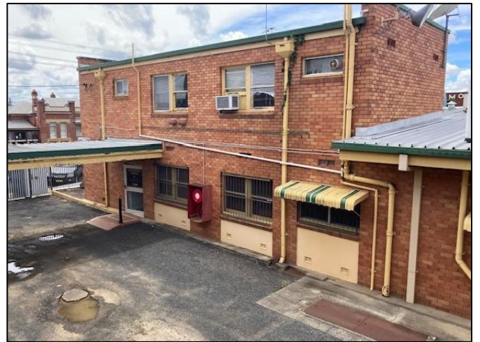
Plate 4: View of Club Building From Motel
