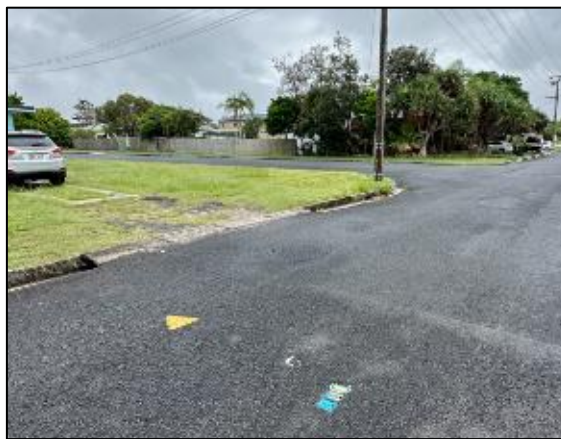
Photo 4: Street hydrant located in Beech Street south of the subject property.
