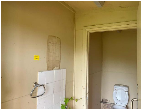
Line ID 46: Internal, Building B, Toilet Rooms, Walls and Ceilings, Beige Paint - Lead Detected (<0.005% w/w)
