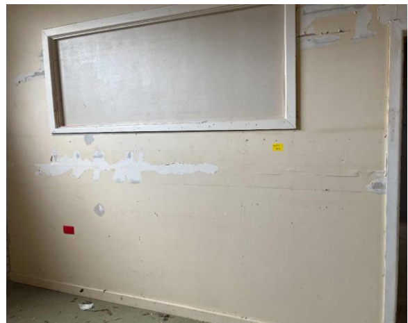
Line ID 43: Internal, Building A, Ground Floor, Eastern Room, Northern and Western Walls, Cream Paint - Lead Detected (<0.005% w/w)
