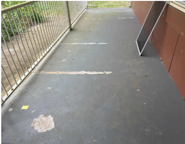
Line ID 38: External, Building E, South Side, Floor, Blue Paint - Lead Detected (<0.005% w/w)
