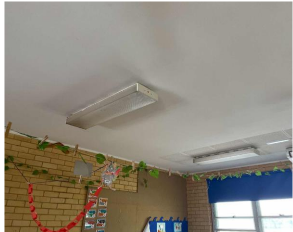
Line ID 61.1: Internal, Building A, Level 1, Throughout, Light Fittings, Ballast(s) - Suspected PCB
