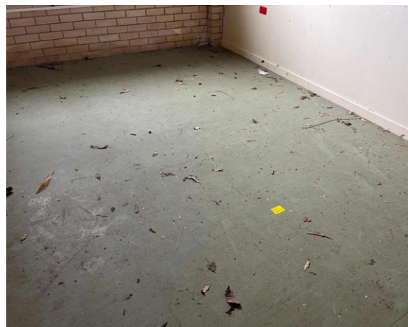
Line ID 18: Internal, Building A, Ground Floor, Eastern Room, Floor, Green Vinyl Sheet - No Asbestos Detected
