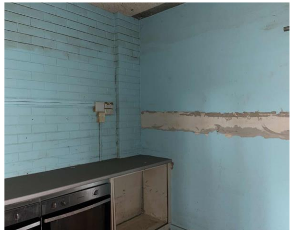
Line ID 41: Internal, Building A, Ground Floor, Canteen, Walls, Blue (Light) Paint - Lead Detected (<0.005% w/w)
