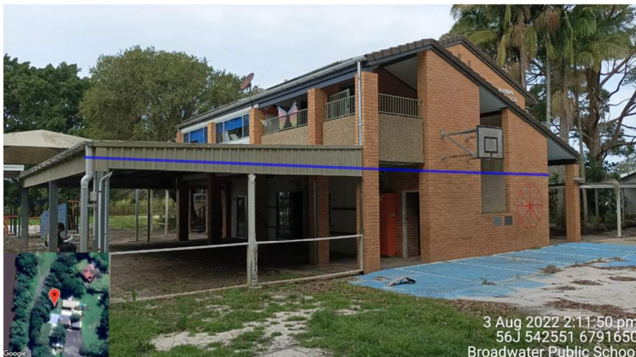
Plate 4-1 March 2022 approximate peak flood level at Block A (Learning Space) denoted by blue line
