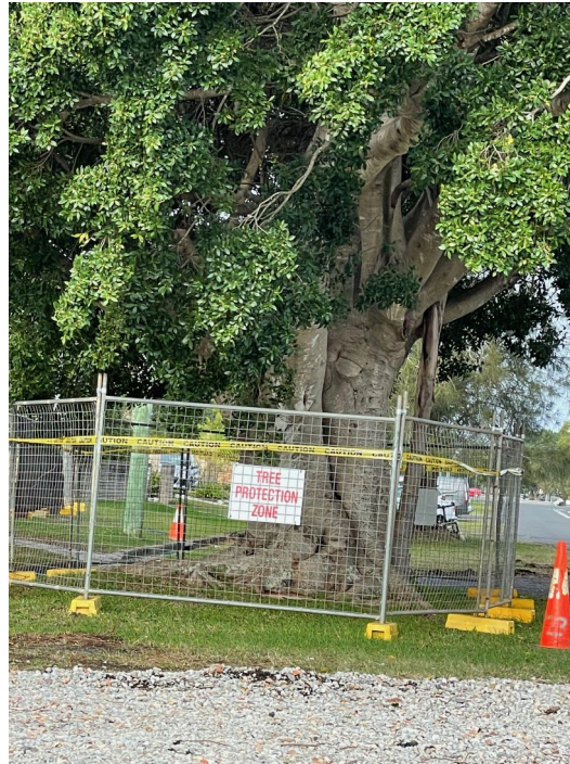
Figure 2. Example of a suitable protective fence
