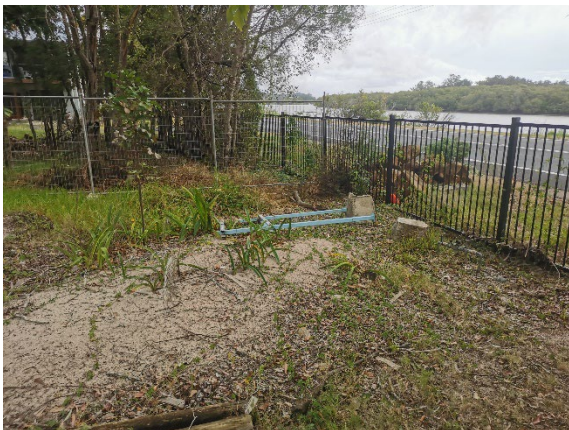
Photograph 5: drainage culvert located offsite in the southwest corner.
