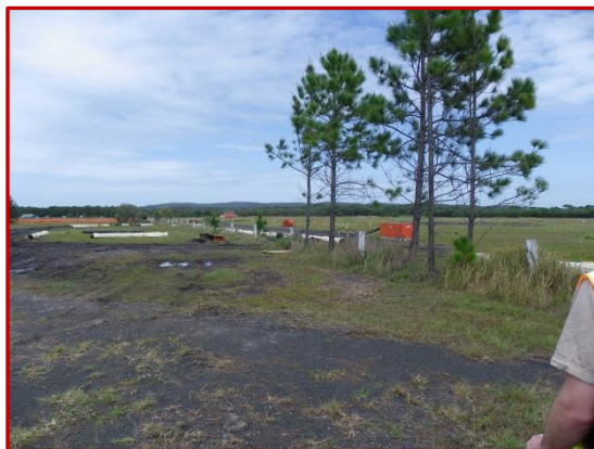
Figure 3.2: The existing fence separating the operational aerodrome (right) with the buffer land next to the residential subdivision.
