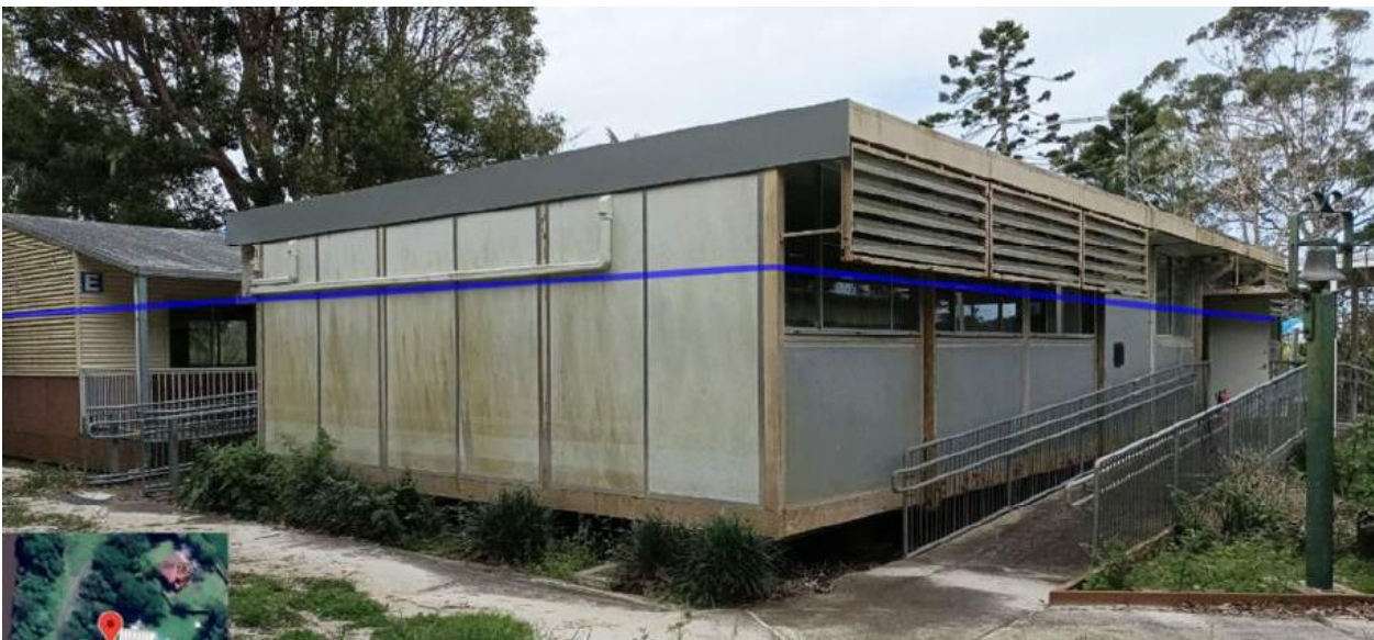
Figure 26: Building D11066 – with Feb 2022 flood height indicated by blue line (Source: Acor Consultants)
