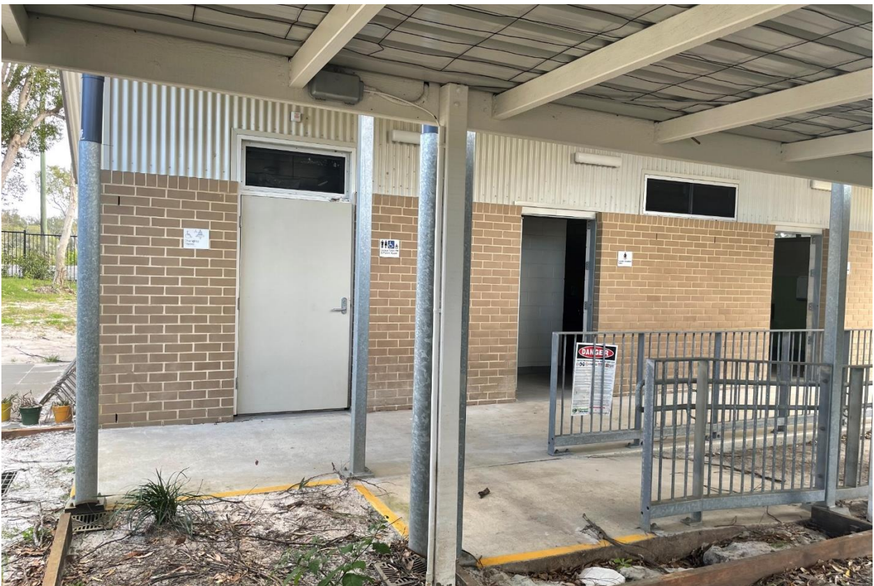
Figure 9: Building J toilet block
