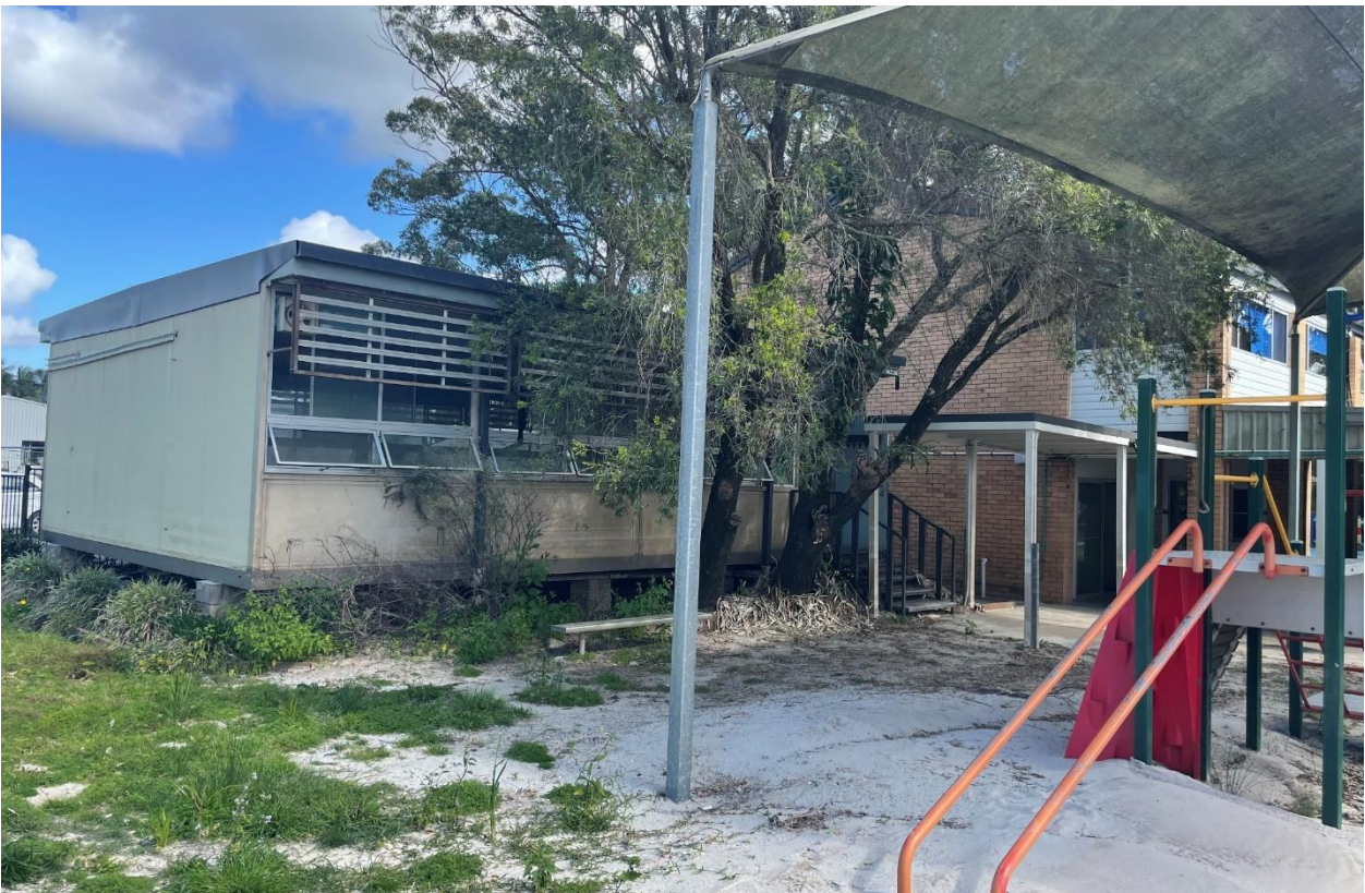
Figure 7: Building D15316 looking south-west towards Building A
