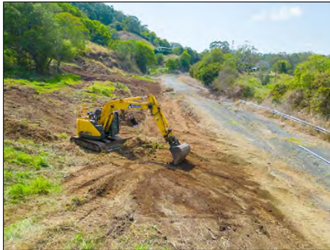
Naughtons Gap Road early works
