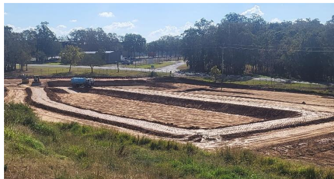
Progress on construction of Cell 6A at Nammoona.
