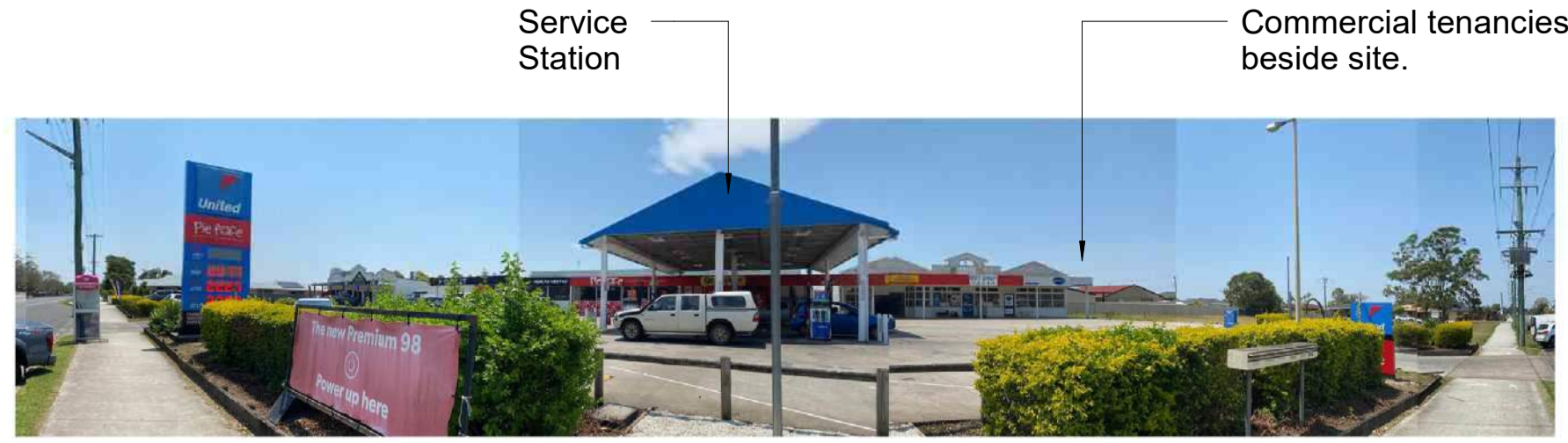
EASTERN ELEVATION OF CLARK ST Adjacent to Site
