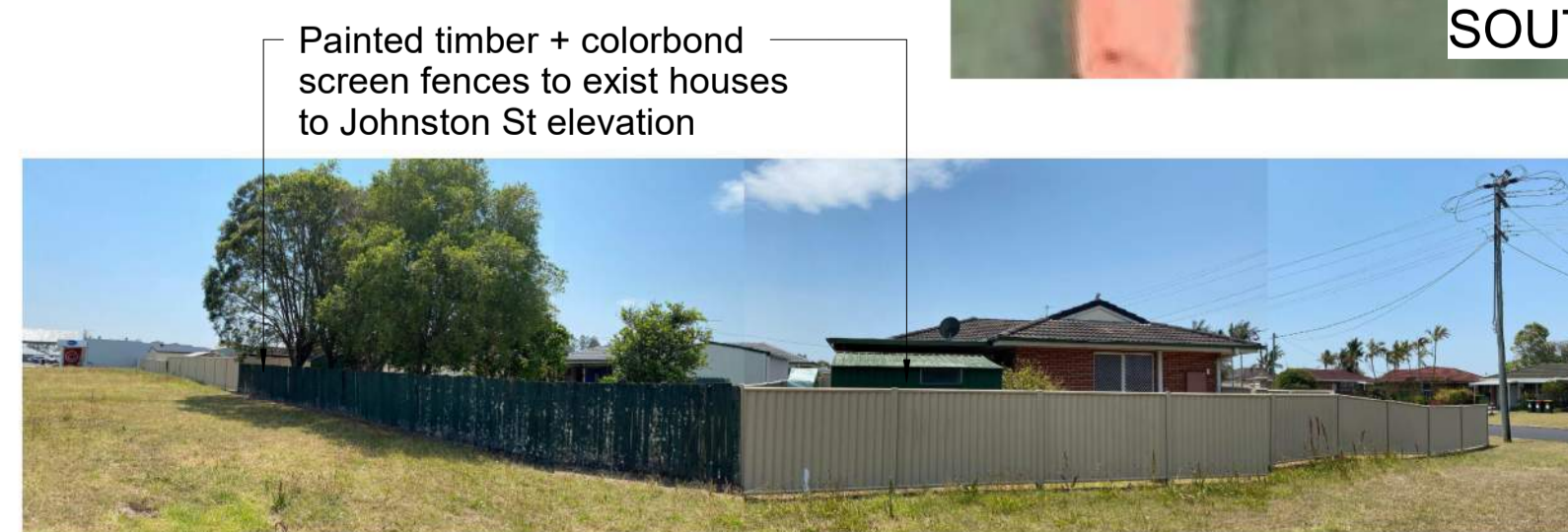
ELEVATION OF SIDE OF SITE (NORTH SIDE) Exist Houses Adjacent to Site
