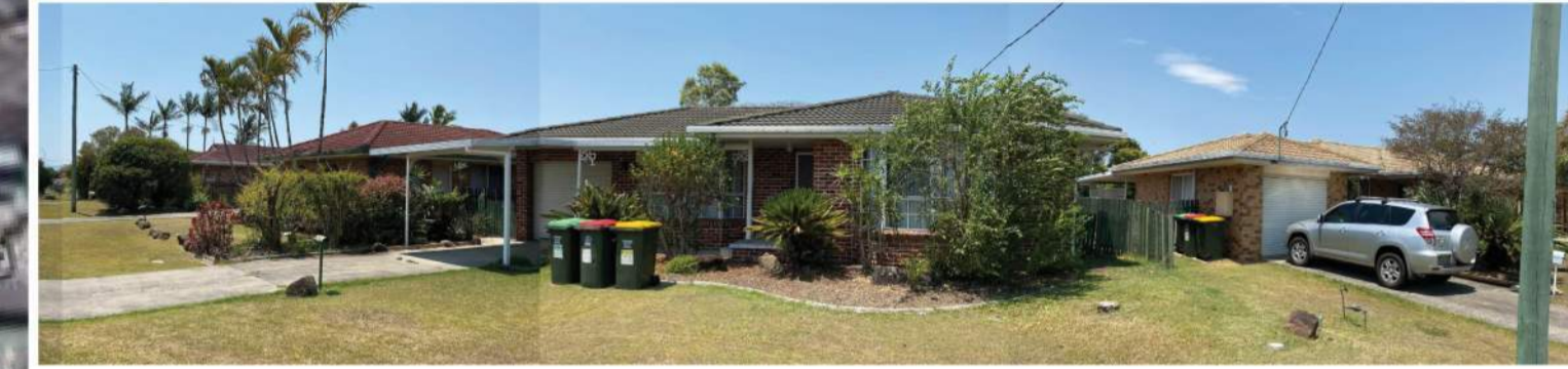
CLARK ST STREETSCAPE Opposite Site (approx)
