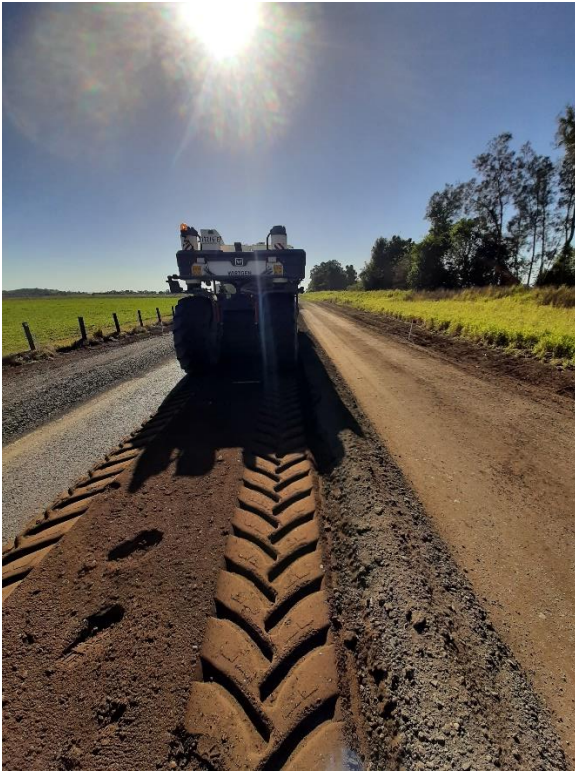
W200 Wirtgen Stabilizer at work
