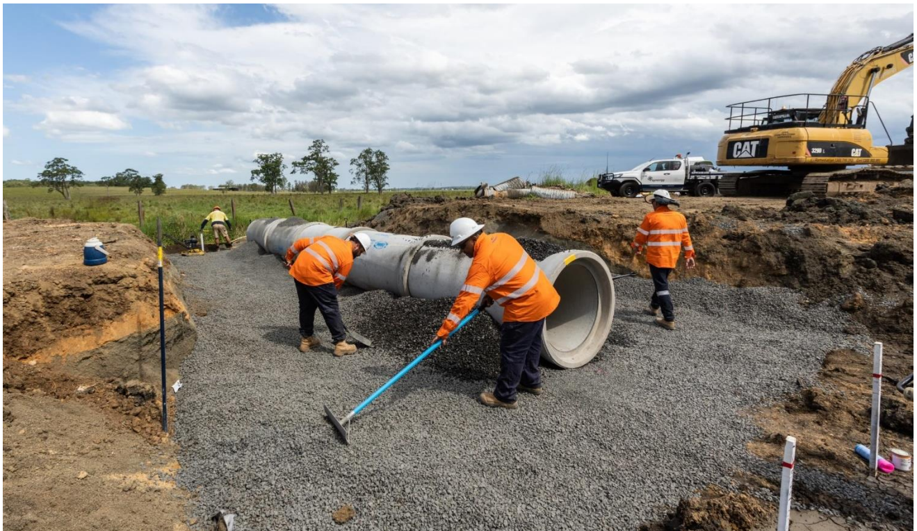
Installing culverts as part of the Benns Rd upgrade
