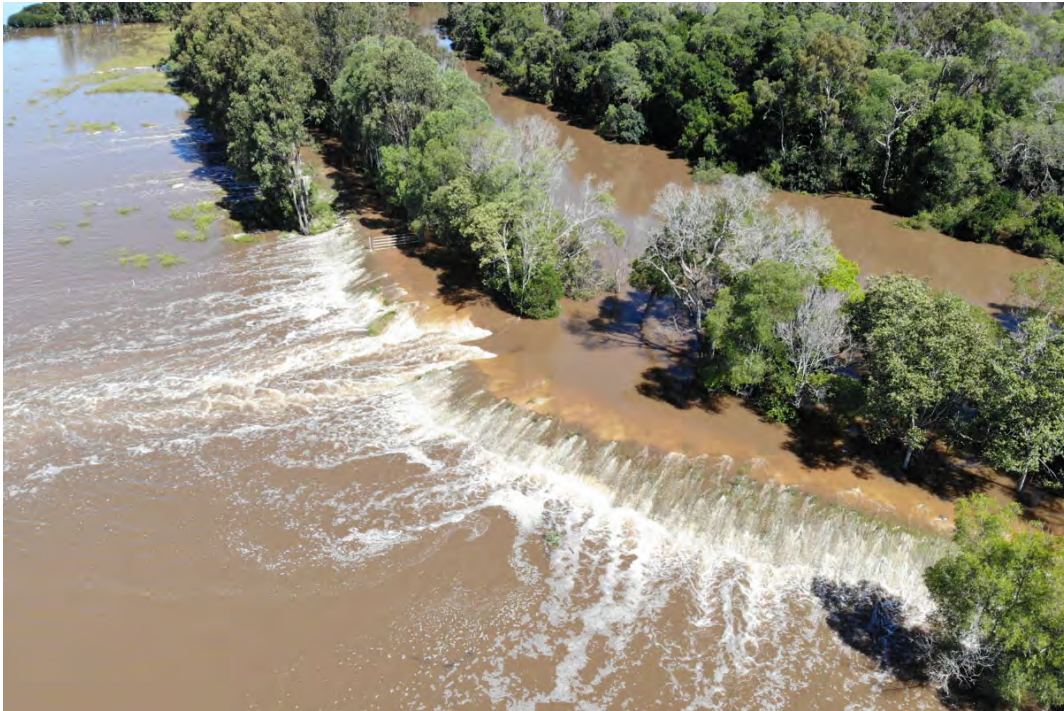
Figure 3.2 Breach and subsequent erosion of levee on lower Bungawalbin Creek (March 2021)
