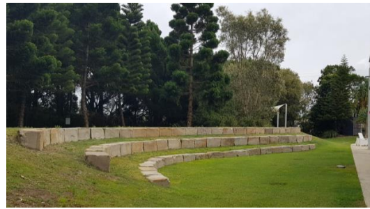
Sandstone block terracing for Woodburn Street bank
