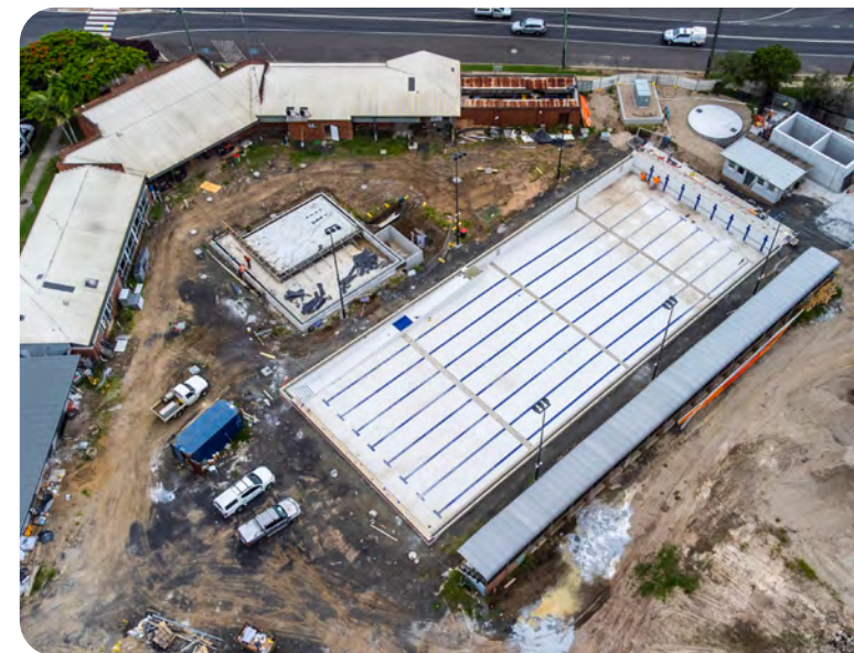
Stage 1 of the Casino Pool upgrade is nearing completion.
