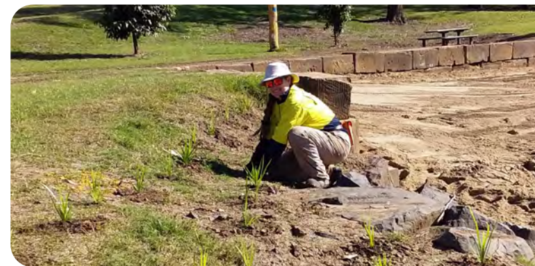
Replanting flood-damaged riverbank at Coraki
