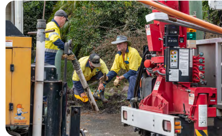
Repairing flood damaged water services in Broadwater
