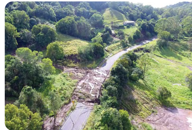
Naughton's Gap landslip repairs will soon be underway
