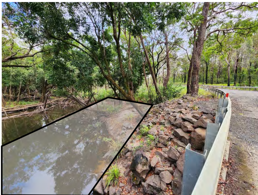
Plate 3 – Temporary steel bridge location – looking north
