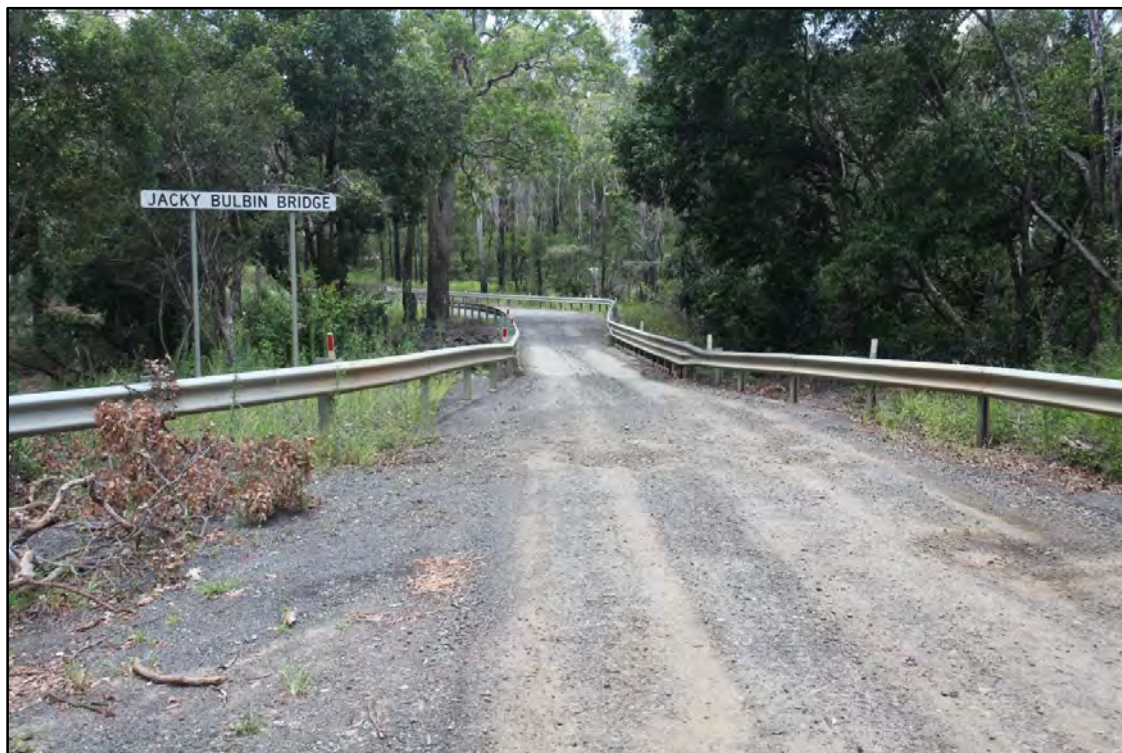
Figure 14: Jacky Bulbin Bridge looking north
