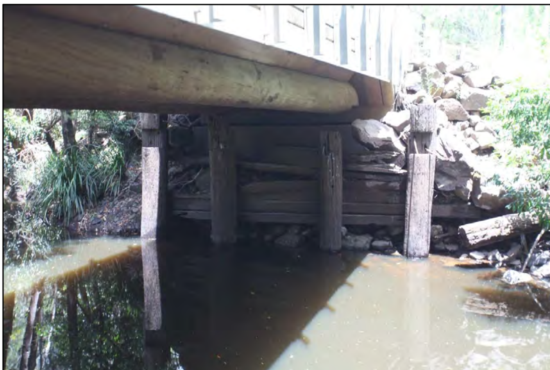
Figure 15: The southern abutment showing original timbers and the current bridge
