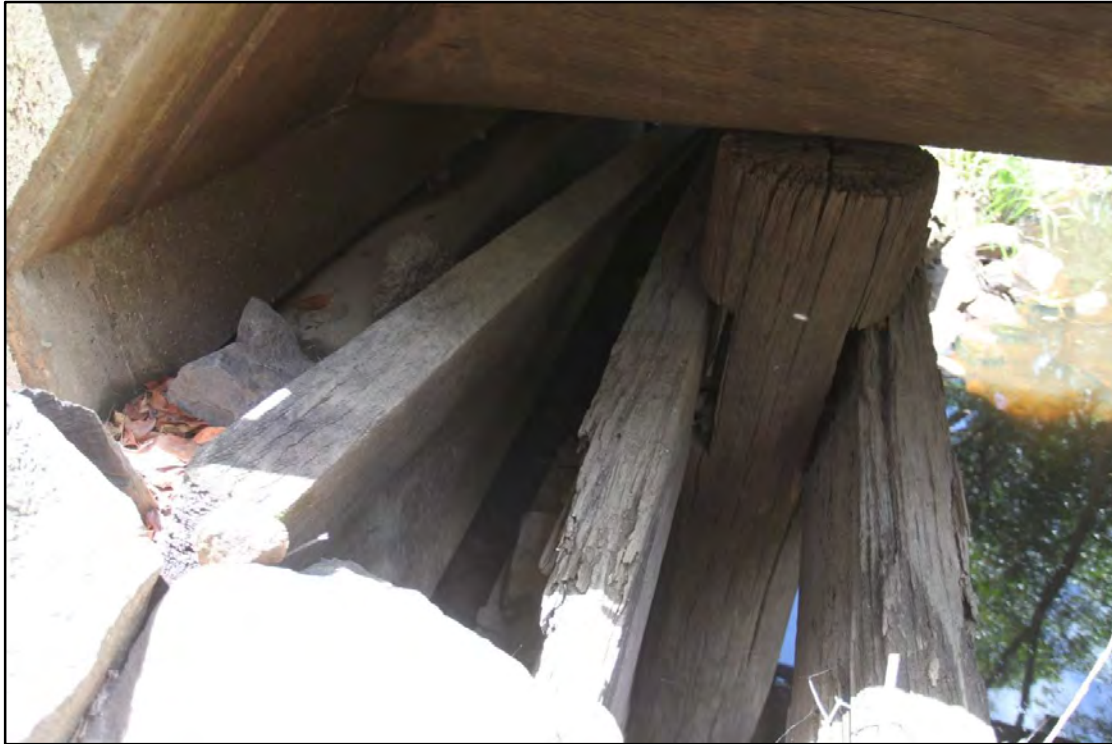
Figure 16: Timber pile and abutment on northern bank with concrete abutment behind
