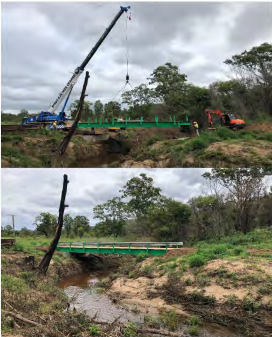
Figure 4 – Temporary steel bridge set up that will be utilised during construction
