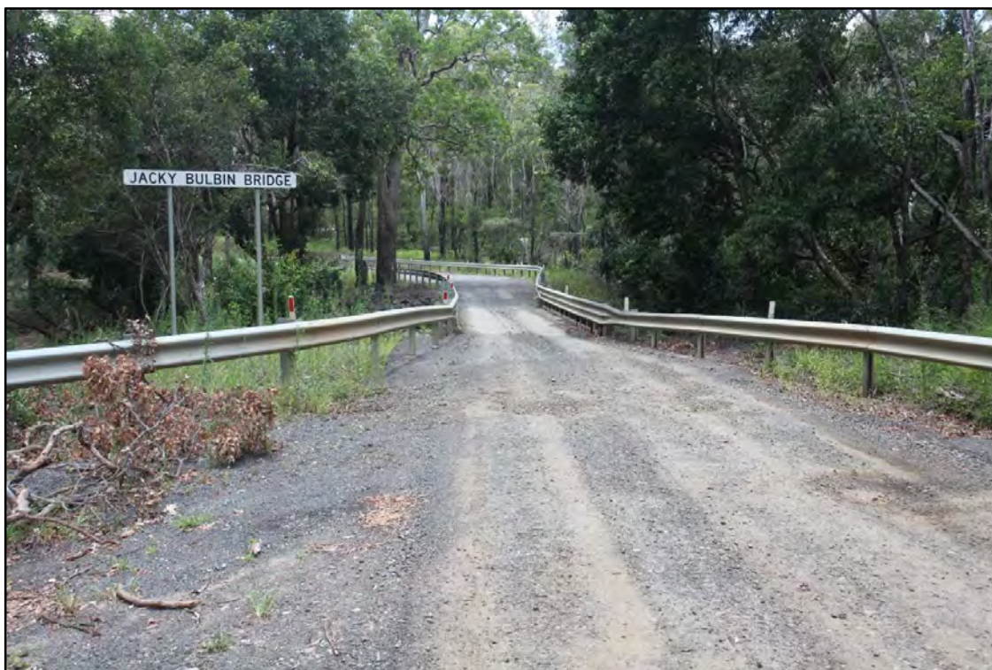
Figure 14: Jacky Bulbin Bridge looking north
