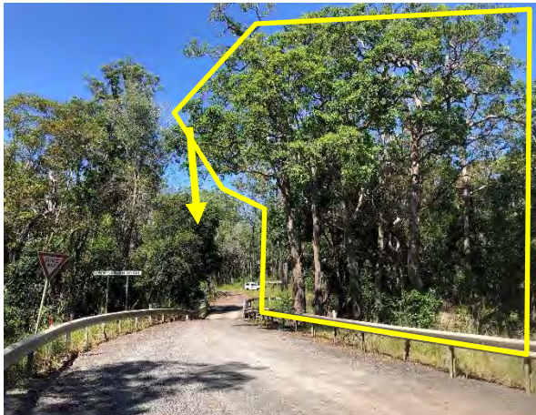
Plate 3.3 View south of Jacky Bulbin Bridge and vegetation west of bridge to be removed (vegetation in yellow polygons to be pruned)
