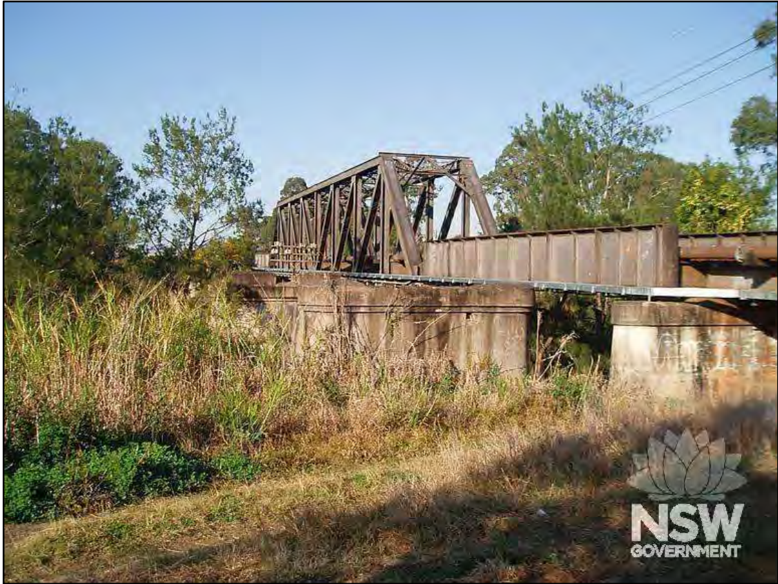
Figure 12: Richmond River Underbridge, Casino
