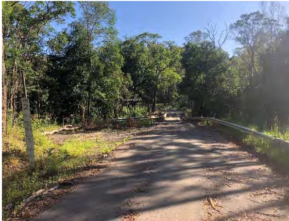
Plate 1.1 View north of Jacky Bulbin Bridge over Jackybulbin Creek
