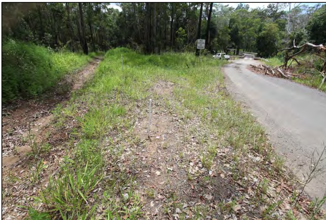
Figure 20: Typical road verge and drain south of Jacky Bulbin Bridge
