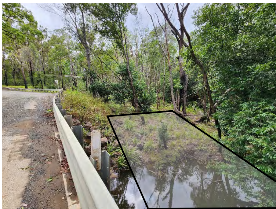
Plate 4 – Temporary steel bridge location – looking south
