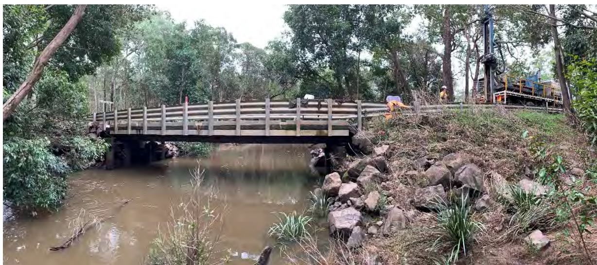
Looking west towards the bridge, drill rig setup at BH1.
