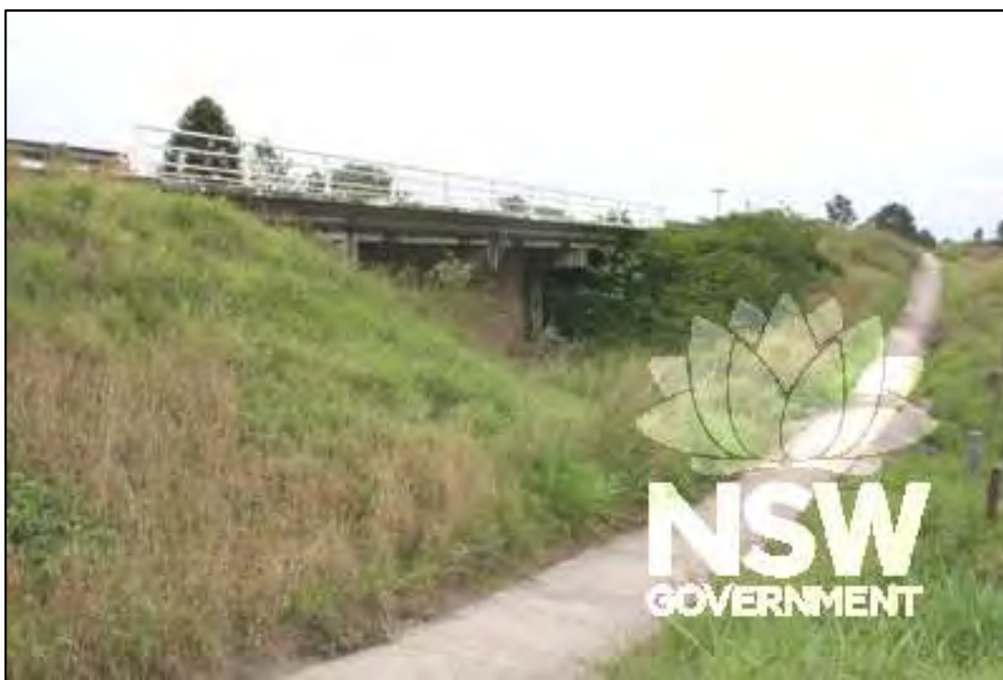
Figure 11: Black Gully Bridge, Casino
