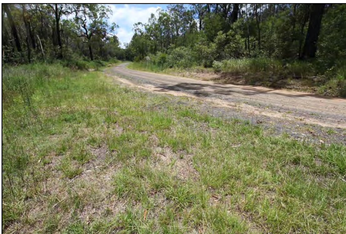
Figure 21: Typical road verge and drain north of Jacky Bulbin Bridge
