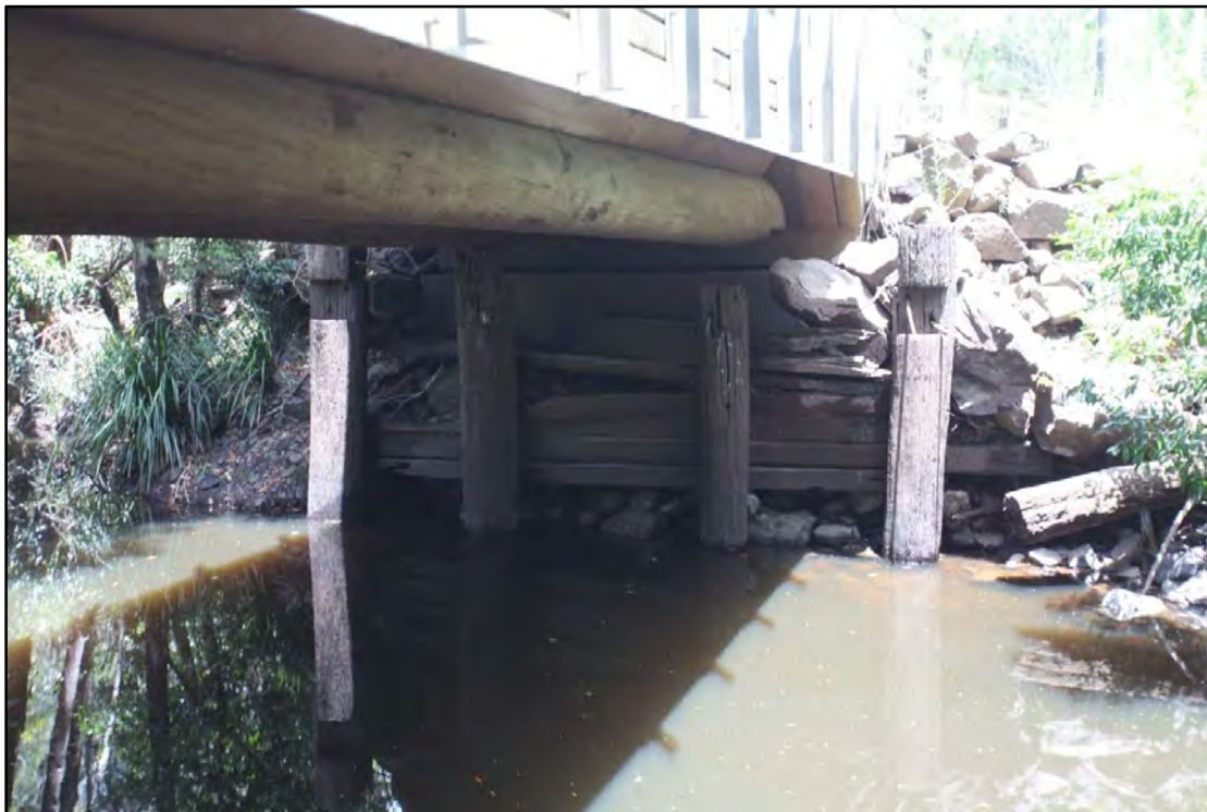
Figure 15: The southern abutment showing original timbers and replacement concrete/ timber bridge
