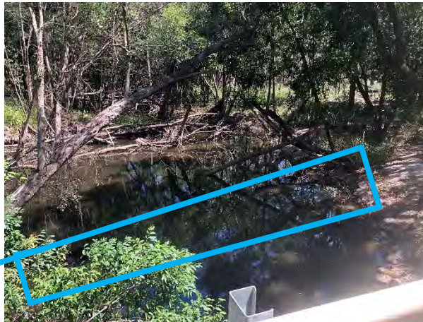
Plate 3.4 View west (upstream) of Jacky Bulbin Bridge (blue polygon indicates new bridge alignment)
