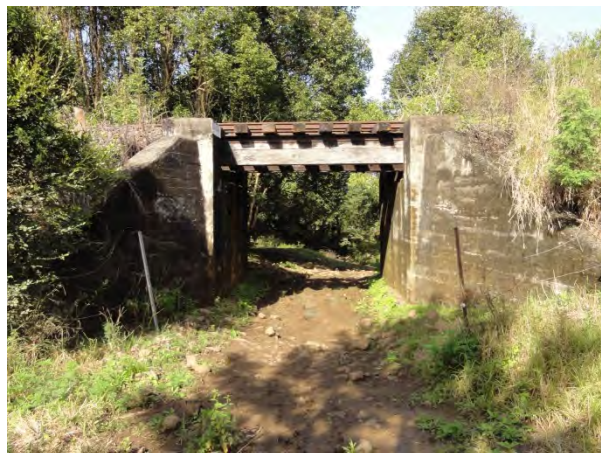
Figure 11 Typical short length underbridge
