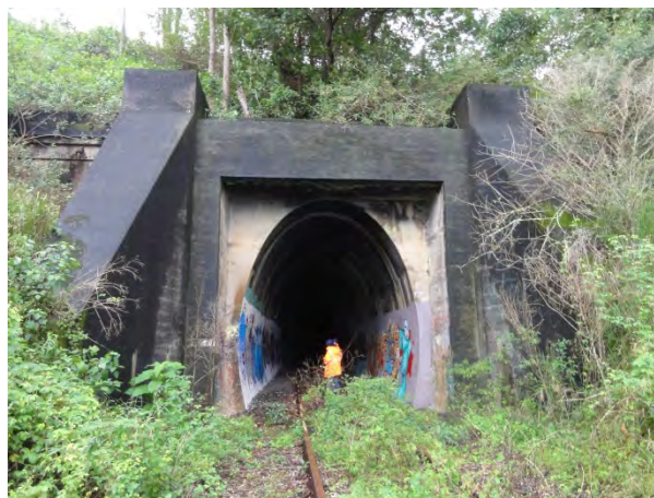
Figure 15 Naughtons Gap Tunnel, TU001 CH815.672km
