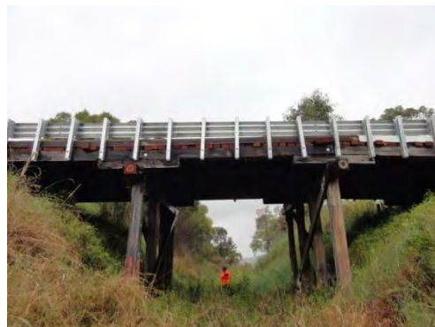
Figure 14 Typical Overbridge, OB001, CH 814.840km
