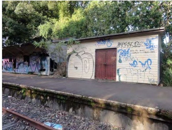
Figure 6 Existing station buildings at Bangalow
