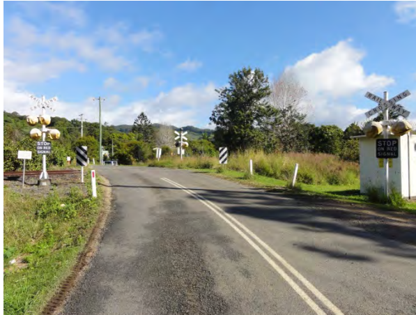
Figure 8 Active Level Crossing - LX097 Upper Burringbar Road CH 919km 539
