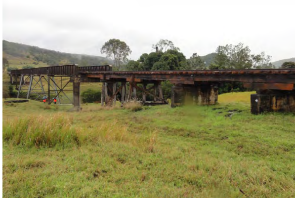
Figure 9 Example of Dual Material Structure, UB027 CH826.684km
