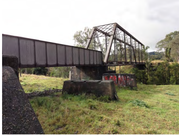
Figure 10 Steel Truss Bridge, UB012 CH819.510km
