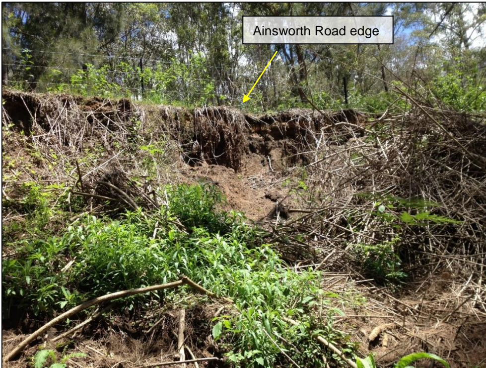
Figure 2: Creek bank erosion adjacent to Ainsworth Road
