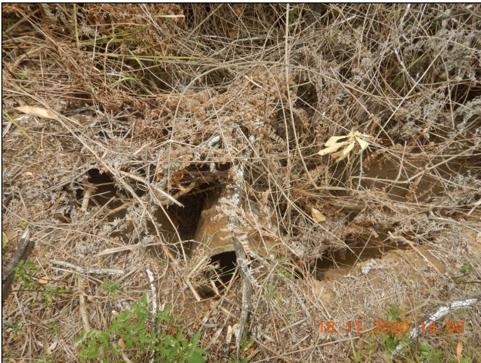
Figure 3: Damaged pipe culvert (downstream outlet)
