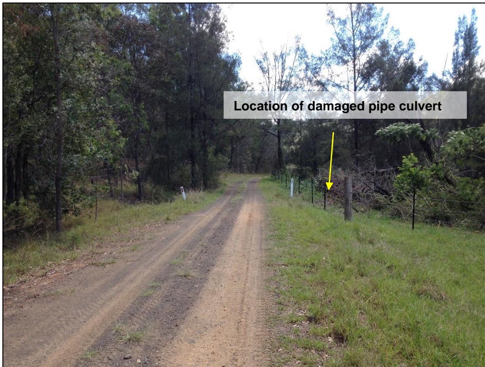
Figure 1: Ainsworth Road. Middle Creek on right hand side of fence
