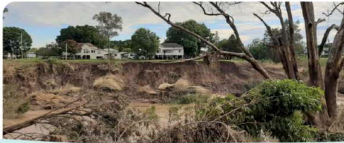
Major riverbank erosion at Casino
