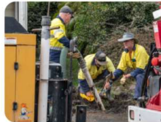
RVC work crews restoring water services at Broadwater
