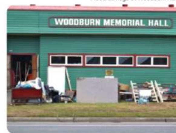
Flood damage at Woodburn Hall
