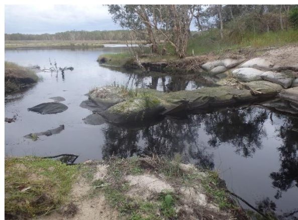
Plate 4.2 The damaged erosion control structure.
