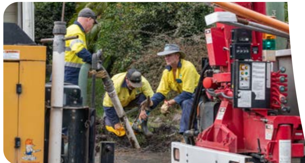
RVC work crews restoring water services at Broadwater
