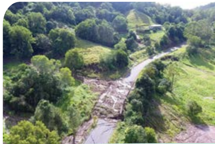
Naughtons Gap Road landslip
