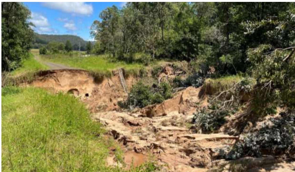
Major wash-away at Upper Cherry Tree Road.
