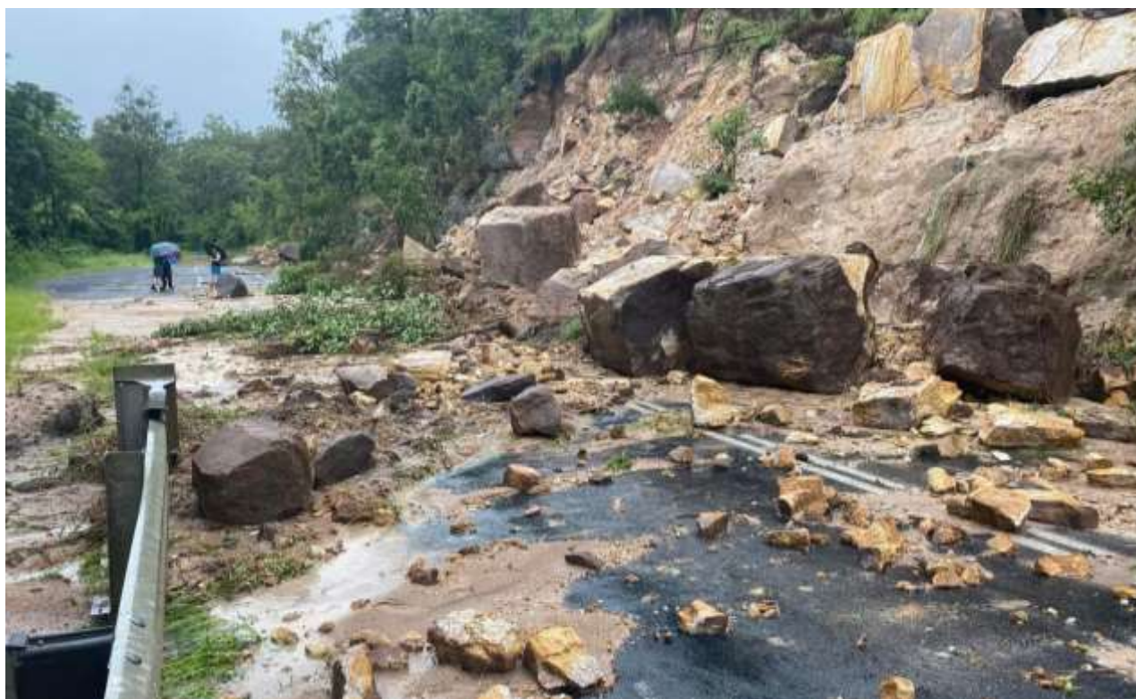
Landslip on Bentley Road
