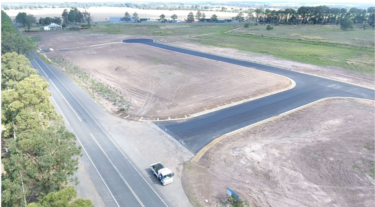
Image 1 – Showing Reynolds Road site roadworks completed.
