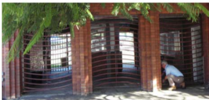
EXISTING METAL GATES- TO BE REMOVED
