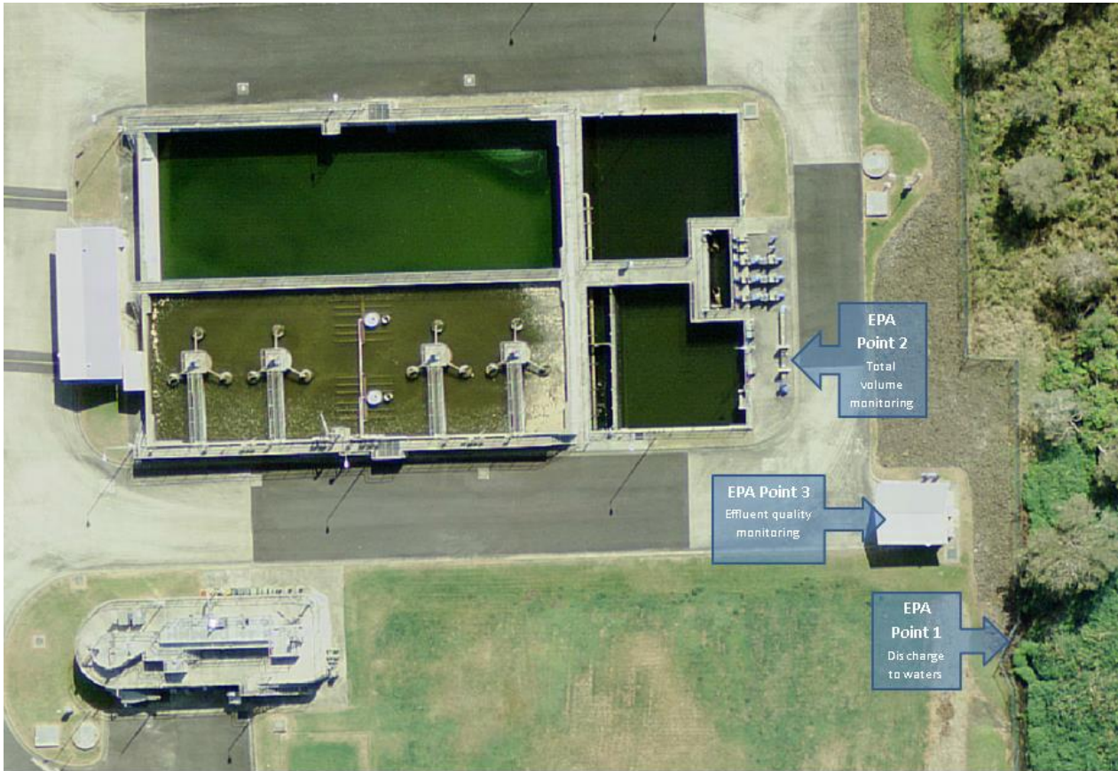
Evans Head Treatment Plant EPA Points
