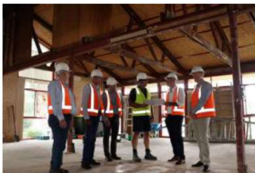
Pictured Above: Inspecting the work progress on the Evans Head Project
