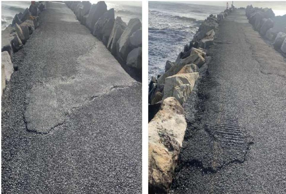
*Southern break wall, damaged bitumen pavement*
