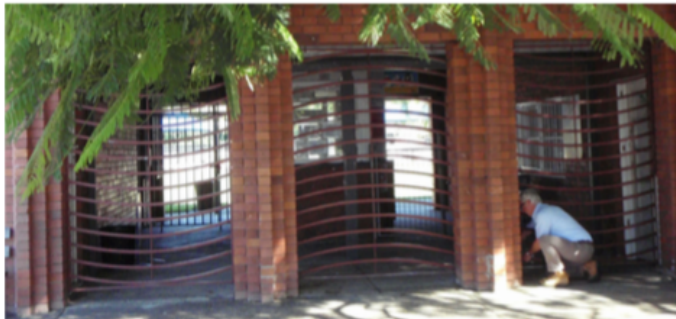
EXISTING METAL GATES- TO BE REMOVED
