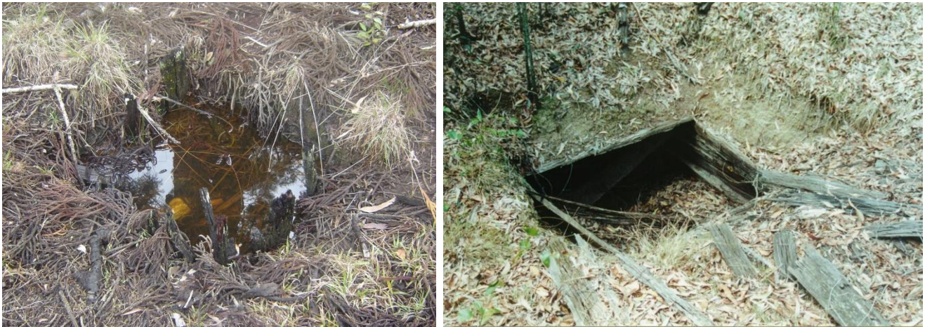
Figure I-16.3 Examples of timber lined wells
