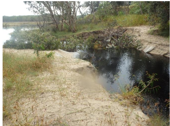
Plate 5.2 Evidence of a reduction in the level of the scour spillway on 30 April 2021.
