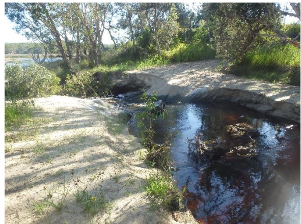
Plate 4.2 Evidence of a slight reduction in the level of the scour spillway installed to reduce the erosive pressure on the head cut.
