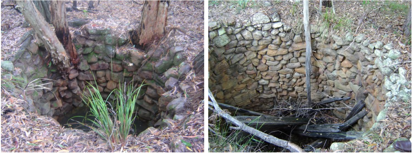
Figure I-16.2 Examples of stone lined wells
