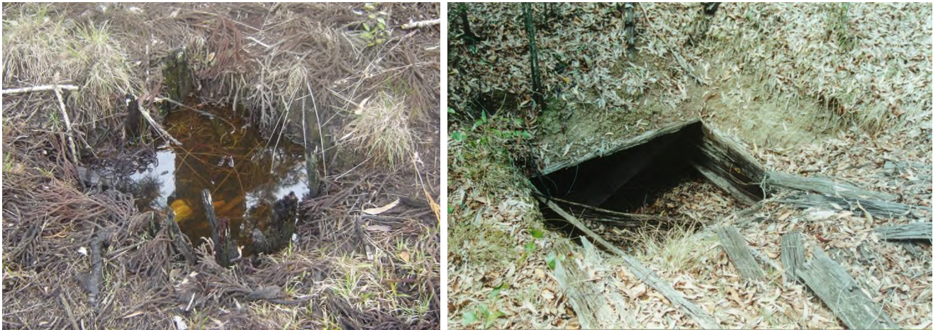
Figure I-16.3 Examples of timber lined wells
