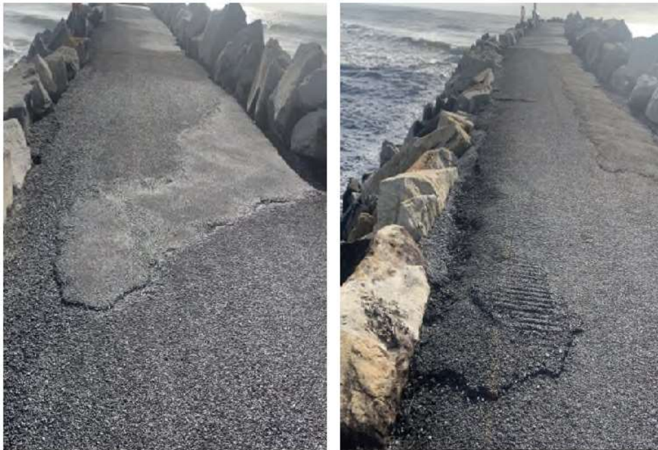
Southern break wall, damaged bitumen pavement
