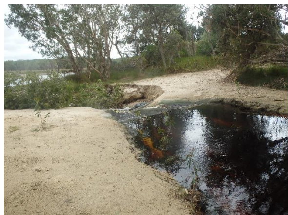
Plate 4.2 Scour spillway installed to reduce the erosive pressure on the head cut.
