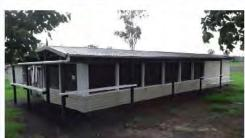
Building - BBQ area Structural shell constructed of timber and weatherboard cladding of very good condition (1.5). Roof constructed of metal of very good condition (1.5).
